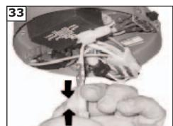
Locate blue and white wire from the fan marked "For light kit". Connect blue from fan to black from light and white from fan to white from light by pushing connectors together.
